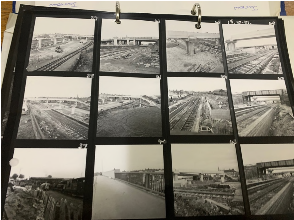
Figure 2- 15.10.1981 showing construction of Hebburn station, note the supports being added for ramp to platform level
