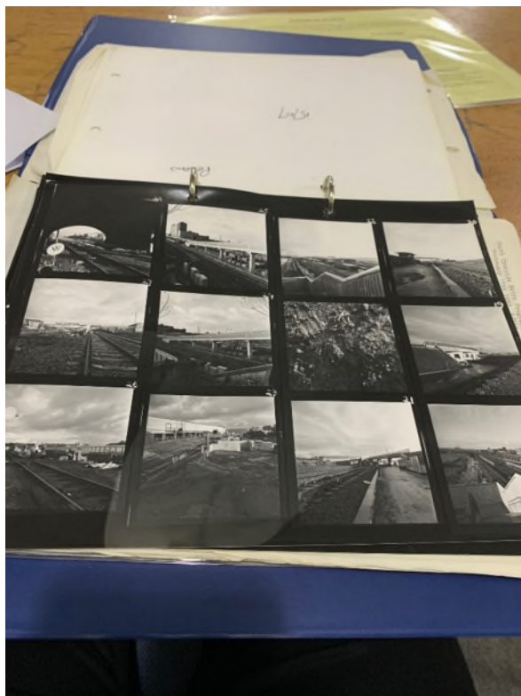
Figure 3- Further shots during construction 1982
