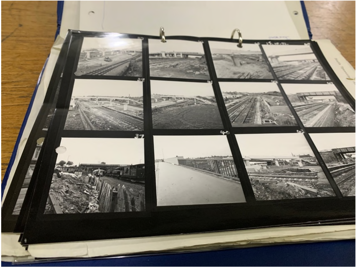
Figure 1- Showing early construction of Hebburn Station for Metro
