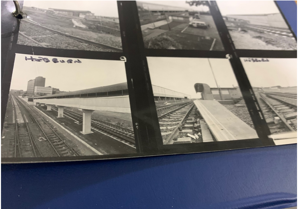
Figure 4- Photos of finished Hebburn Station both Platform 1 and 2
